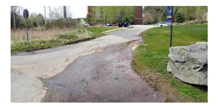
On a related but separate note, we have identified an area of calcium carbonate leachate that has entered a nearby wetland in an area to the south of the Greggs Hall access road. It appears that due to the installation of the duct bank, calcium carbonate from the flowable fill has leached from soils on the south side of the access road and entered a cattail swamp in this area.
