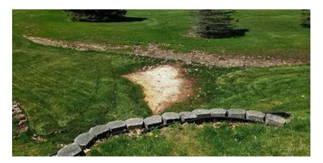
In the area of the Veitas property located at Gundalow Landing in Newington, it appears that the drainage patterns have shifted and a white precipitate from groundwater seepage has accumulated over time on the sod in an approximately 10 x 20 ft area above the cable duct bank (which is also in the vicinity of a stormwater culvert). Eversource has removed the precipitate from the ground surface and we are monitoring the area.
